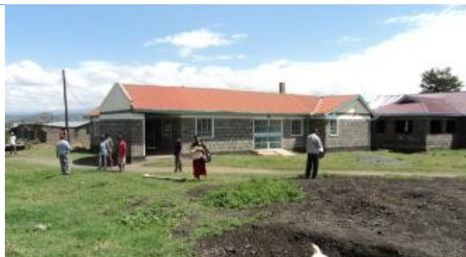
12. Rhonda dispensary under construction
