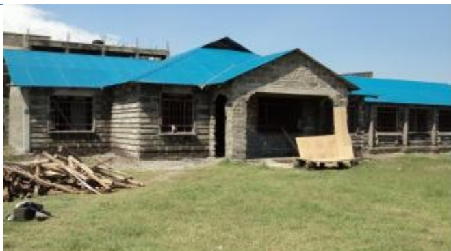
9. Langa Langa health centre general ward under construction
