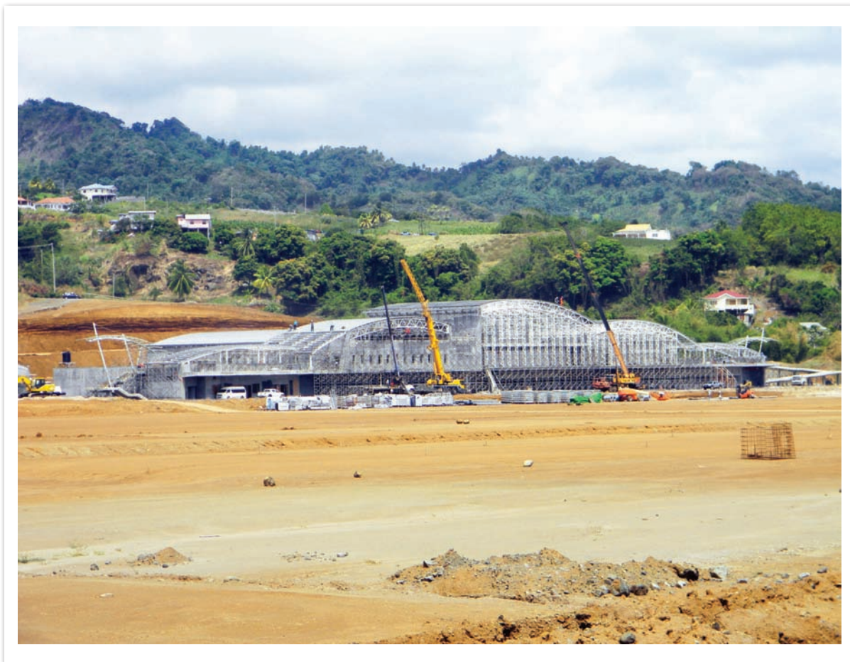
Photo 5.1: Construction Site - Argyle International Airport
