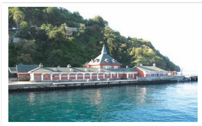
Photo 5.13: Cruise Ship and Ferry Berth, Kingstown
