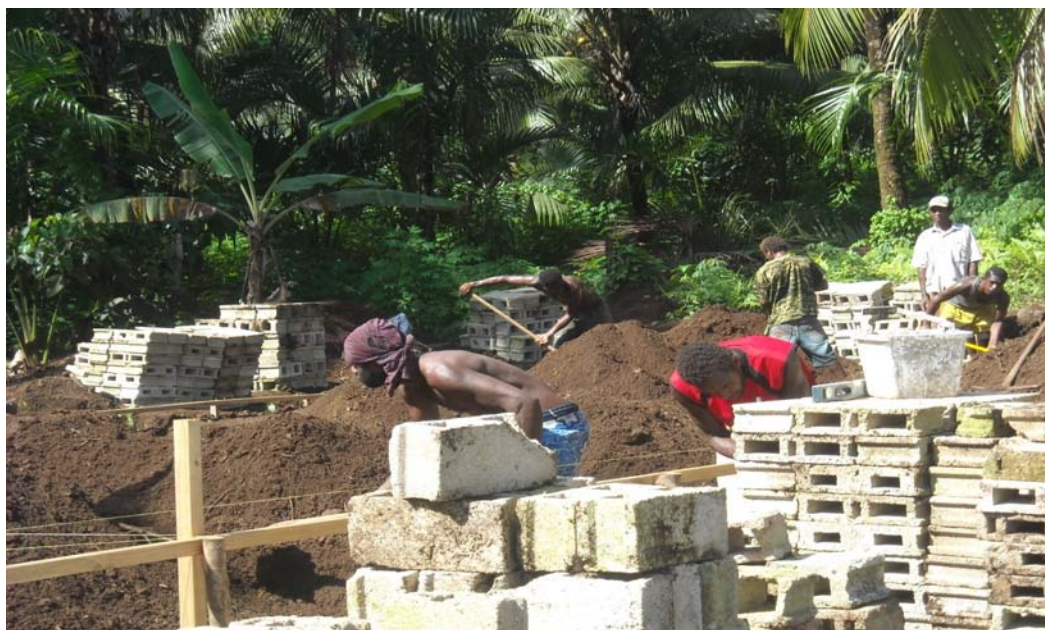
Torba Mini- Hospital Construction: Part of MOH health infrastructure development
