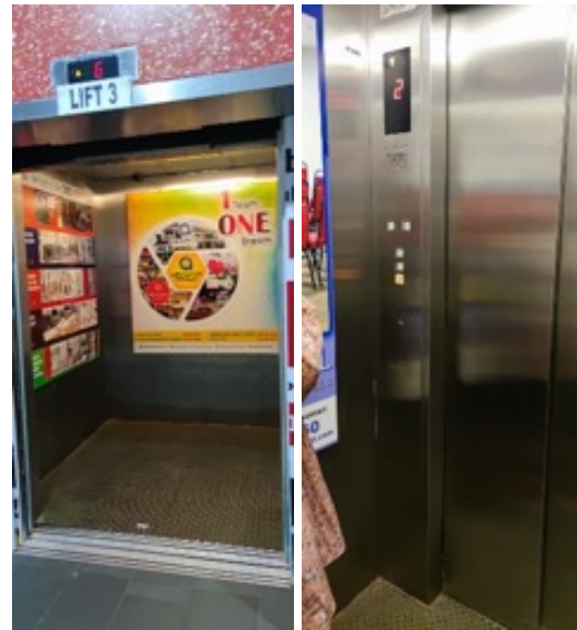
Picture 4.1: Observed lifts in Taiping Central Shopping Complex, Taiping, Malaysia
