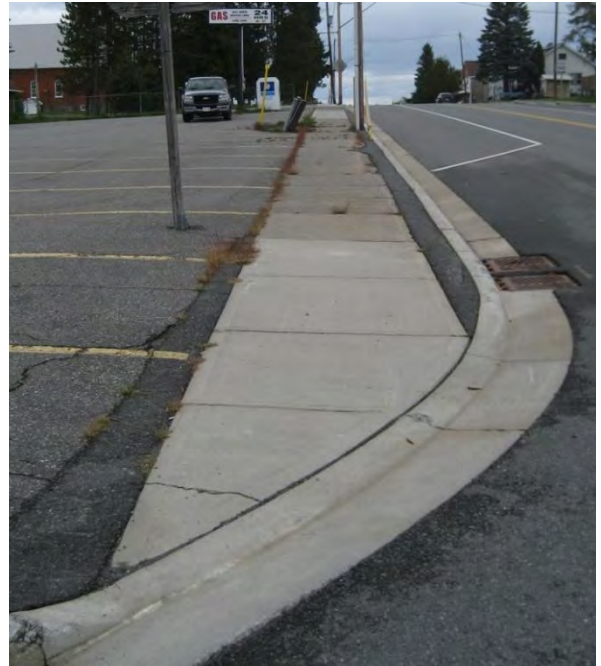
Level sidewalk and dropped curb provides easy access for mobility device users.
