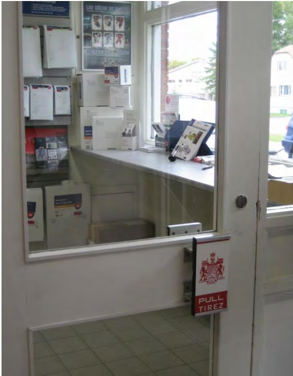
Standing-height counters at public buildings may be difficult to access for clients using mobility devices.
