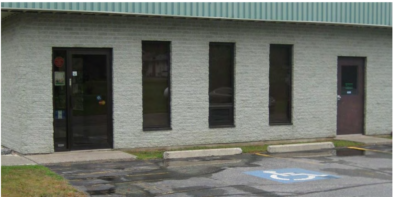
Accessible parking marked only on pavement may not be visible under snow cover.
