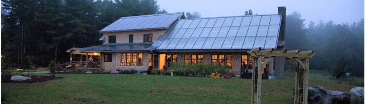
Albany location of Tin Mountain Conservation Center with zero-energy building design
