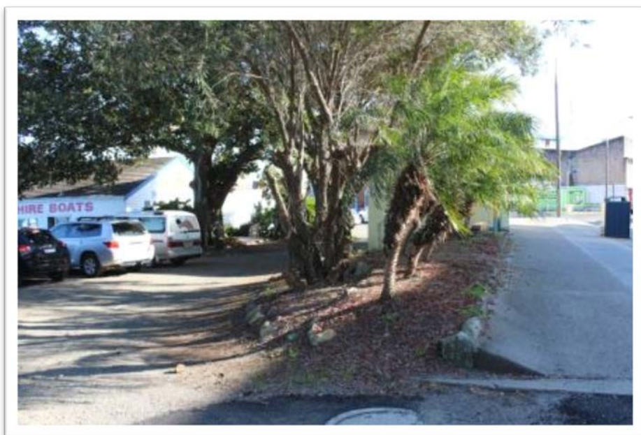
Before - the Little Street bus stop area, showing uneven ground and a dark and dingy area before (with the yellow bus stop structure just visible behind the vegetation on the right). The ground is uneven, vegetation makes lighting uneven, and the carpark increases risk of a reversing car hitting a pedestrian
