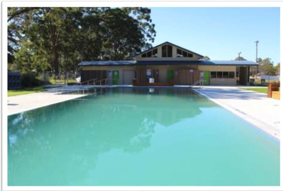
The newly-completed swimming pool at Nahiack
