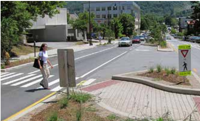
Pedestrian refuge islands buffer pedestrians from traffic, allow crossings in stages and angle pedestrians correctly to face traffic.
