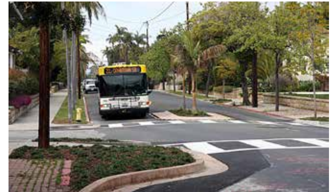
A large vehicle being deflected through a neighborhood Intersection Chicane, Santa Barbara, CA
