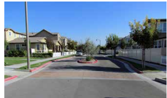
A short median in Loma Linda, CA announces the entrance to a residential neighborhood
