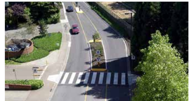
Crossings must be located where there is a strong desire to cross and where sight distances are good
