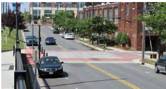
Raised intersections bring speeds under control and help motorists and pedestrians see each other in Birmingham, AL.
